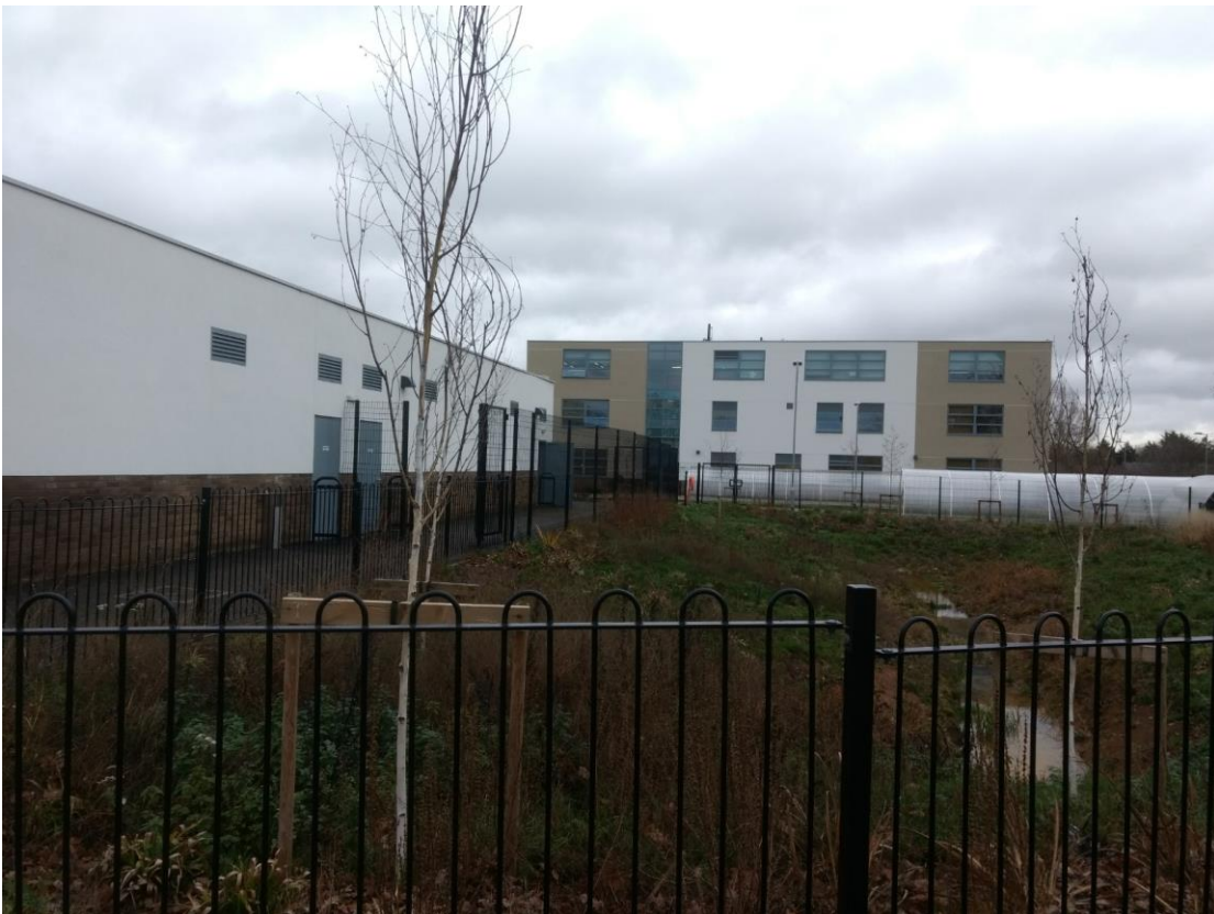
View of front elevation of Sports Block and west elevation of School Block
